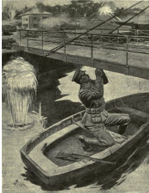
Lance-Corporal Jarvis preparing to destroy a Bridge.
